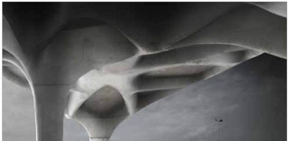
Detail of the structural ribs
