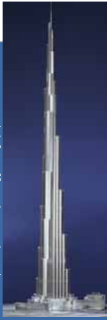
Burj Dubai, designed by and copyright to Skidmore, Owings and Merrill LLP, model photo by Steinkamp-Ballogg Photography.
